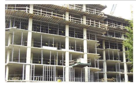
Heavy Duty Post Shore provides the contractor with a safe, light weight, high capacity, easier to use Post Shore. Heavy Duty Post Shore have a much greater capacity than average 20kN Euro type shores. This allows more space between the posts to open up areas that are normally blocked up with shoring equipment. This saves time in erecting, rental dollars in equipment, and makes a safer "trip free" area for workers.
