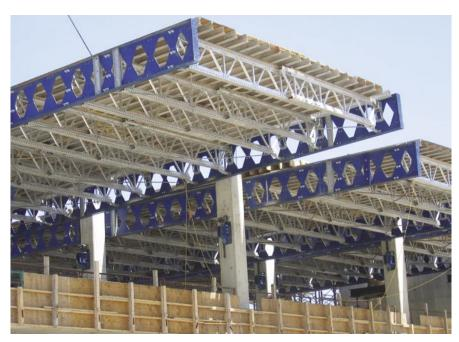
The Hi Flyer® makes reshoring unnecessary. Our heavy-duty Screw Jack simply bolts to the column, which transfers the load down through the column structure itself rather than to a slab below. Follow-up trades can start to work sooner and building materials can be moved in by crane a few days after the concrete has been poured.
