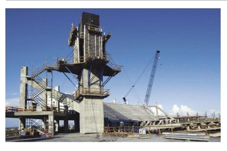
Kiewit Western Co. used the Aluma Systems Wide Platform Rollback to form one of the stadium's 178-foot super columns, which provides primary support for the steel truss roof.
